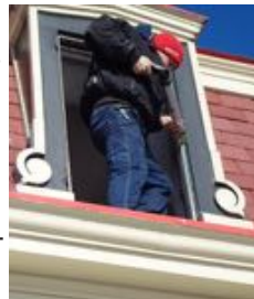
Putting in new storm windows
